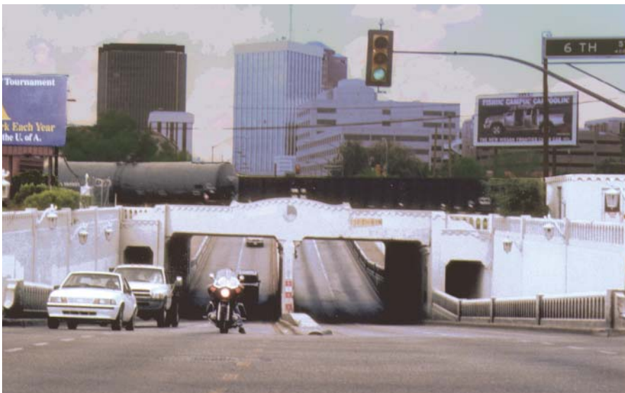
This view along Stone illustrates the corridor's historic linkage to the Downtown from the north.
