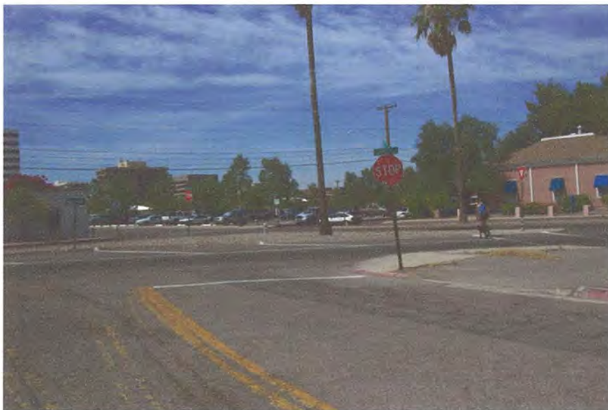
Existing: 9 th Avenue north of Franklin Street looking toward the intersection of Franklin Street and Church Avenue. Note the gravel-filled raised island blocking passage of pedestrians and bicyclists. This project would provide ADA curb cuts and additional sidewalks across the island, allowing more direct connection to the intersection of Franklin Street and Church Avenue for users heading downtown along 9 th Avenue from the Dunbar-Spring Neighborhood.
