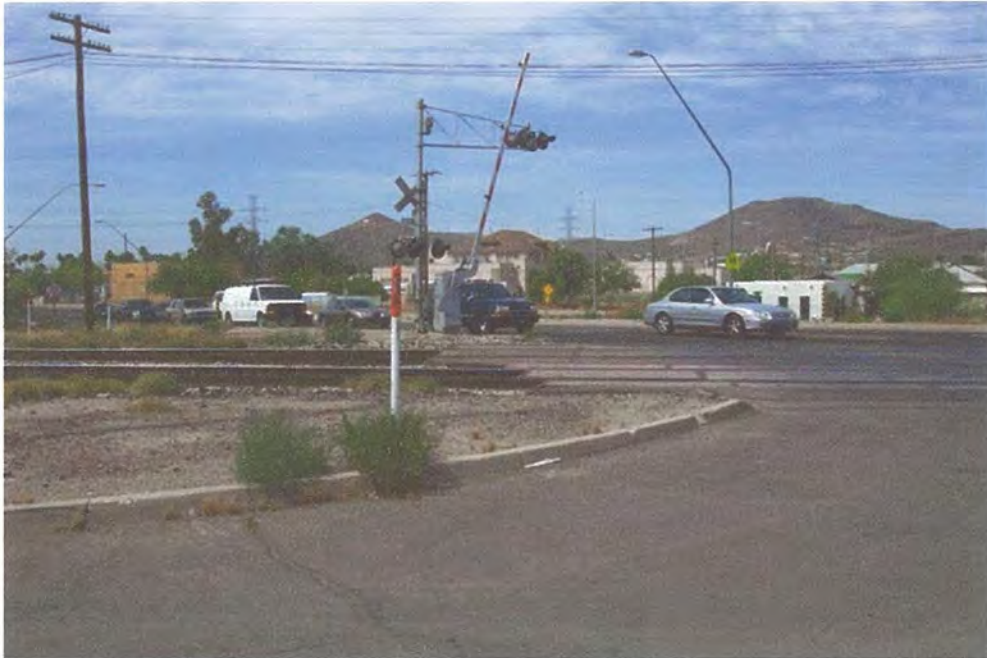
Existing: Looking south from 4 th Street. Missing ramp and sidewalk south of 4 th Street on either side at the Union Pacific Railroad tracks on east side of Main Avenue, westerly edge of Dunbar-Spring Neighborhood, and eastern edge of Barrio Anita Neighborhood.
